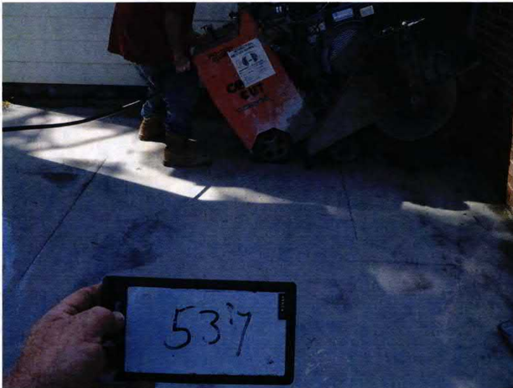
Picture 1: Location of UST 537LaurelBB.
