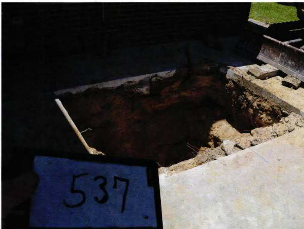
Picture 2: UST 537LaurelBB excavation.
